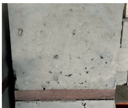
Photo 1. View of the composite specimen: a damping mortar layer with rubber granulate (15 mm, red) and a structural concrete layer (135 mm, C35/45 XM2).
