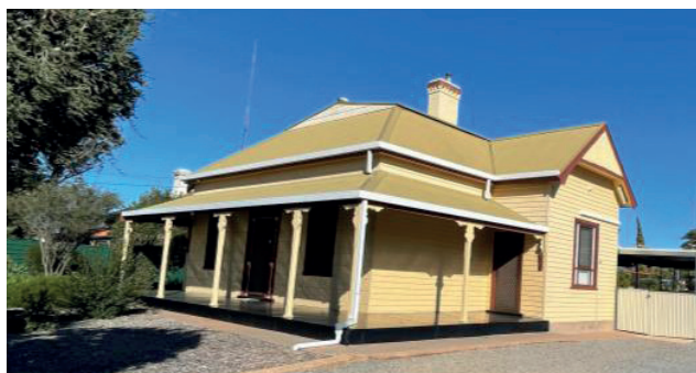
An example of a typical single-family building participating in the research
