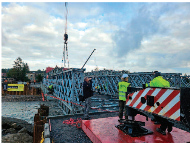
Photo 1. Setting up spans of a crossing made of DMS-65 structures in Glucholazy after the flood in 2024
