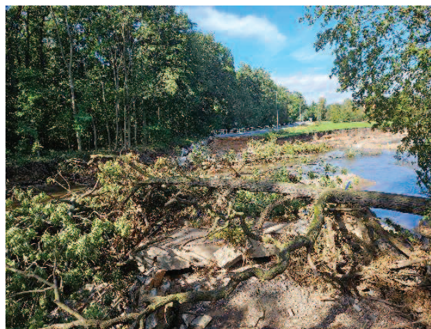
Photo 2. Riverbed 53 m wide; before the flood wave passed, the bridge was 12 m wide – Żywocice
