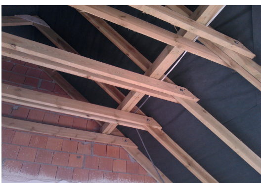
Photo 2. Trusses with two-branch collar beams without support of a queen post wall
