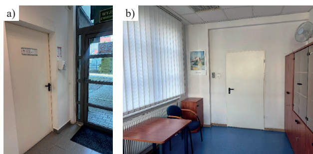
Photo 2. Localization of the source of unstable noise (round II) – view: a) from outside; b) from the office room
