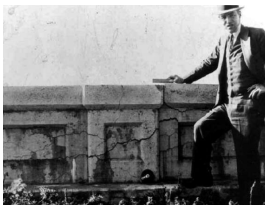
Photo 1. Thomas Stanton in front of a bridge structure affected by alkali-silica reaction [2]
