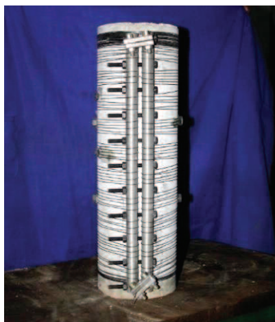
Photo 1. Strengthening of the column with NiTi wires in studies by Hong et al. [22]
