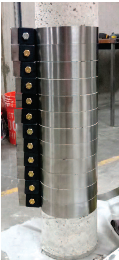
Photo 2. Strengthening of the columns with Fe-SMA strips in studies by Zerbe et al. [15]
