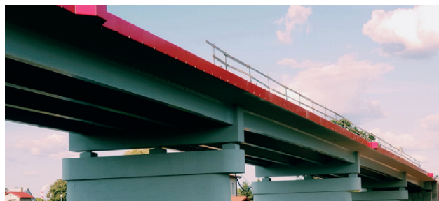
Photo 1. Multi-span composite structure with the girders made continuous by means of concrete support cross-beams
