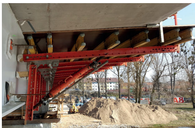
Photo 3. Typical support structure for the formwork of a deck slab cantilever
