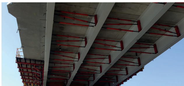
Photo 2. Typical bracing system of main girders – only vertical anti-rotational bracings between girders are applied
