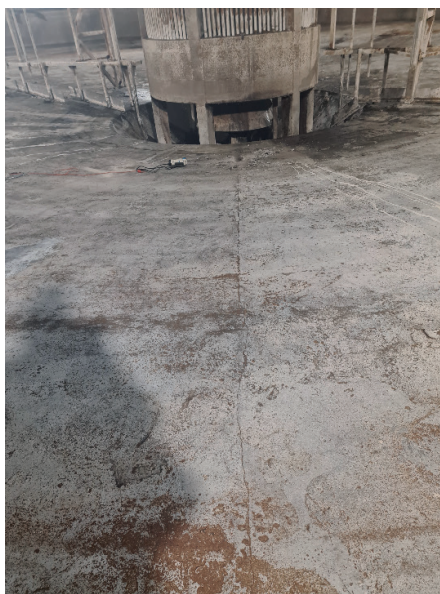
Photo 1. Municipal sewage tank during the third repair of the protective coating
