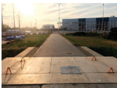
Photo 2. Experimental road section for carrying out vibration damping tests
