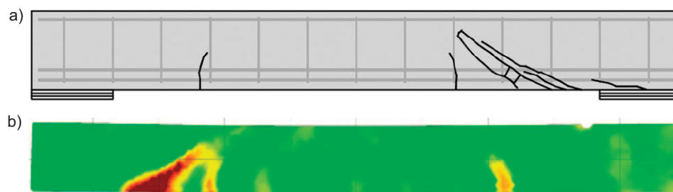
Fig. 5. Cracks of the ND-1 model: a) rear view; b) front view obtained from the Aramis system
