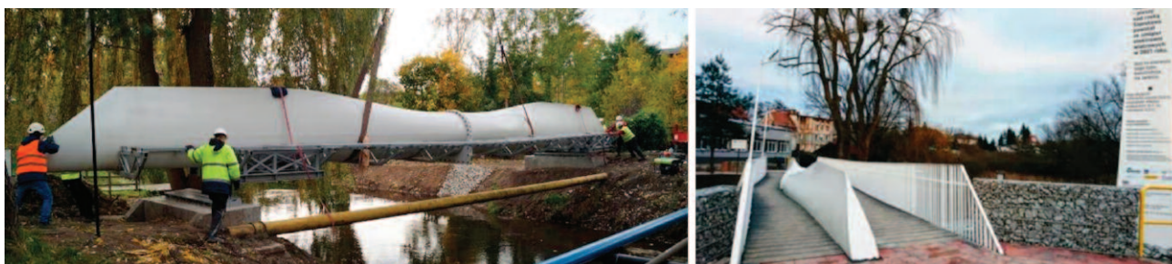
Photo 2. Footbridge in Szprotawa (Poland) [10]
