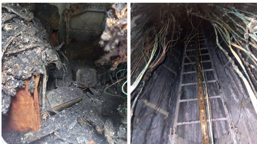
Photo 4. Structural condition of the mast base after dismantling
