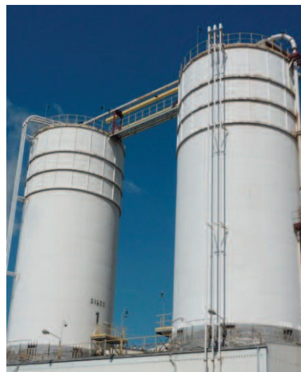
Photo 6. Ring-reinforced silos
