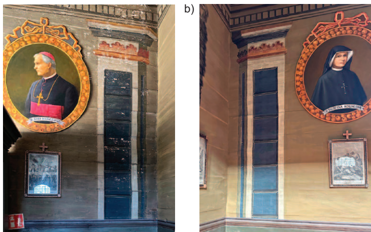
Photo 6. Polychromes; status as of March 2024: a) in the right side aisle before renovation; b) in the left side aisle after current renovation
