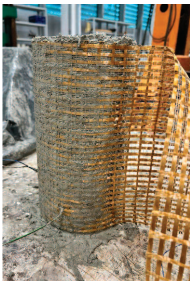
Photo 2. Application of PBO-FRCM composite reinforcement
