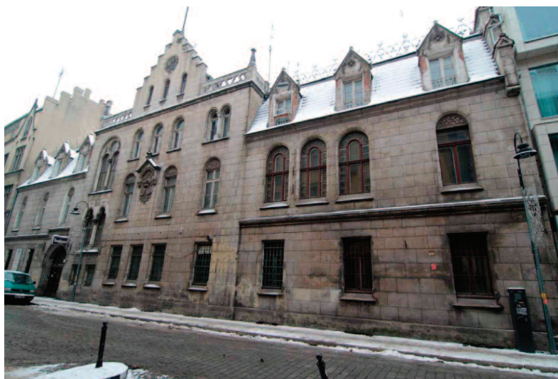
Photo 1. Front façade of the Ballestrem Palace at 4 Włodkowica Street in Wrocław (view before renovation)
