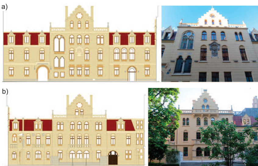
Fig. 3. The façade of the Ballestrem Palace after renovation: a) northern façade (visualization and actual condition); b) southern façade (visualization and actual condition)
