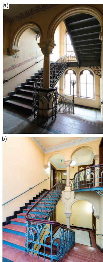
Photo 2. Representative staircase: before (a) and after (b) revalorization
