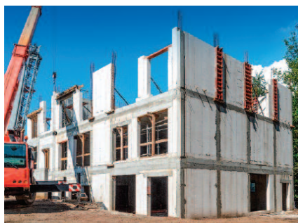
Photo 1. Construction of a kindergarten in Bytom using modular AAC panels
