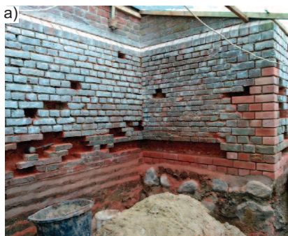
Fragment of the Gothic wall: a) restoration work by the use of currently produced brick; b) after conservation work
