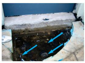
View of the of the polymer-modified asphalt thick coating at the threshold of the door leading to the terrace, with traces of local thickness reduction. The arrows show examples of areas of coating thickness reduction in the region of increased local, pressure
