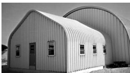
Fot. 5. Obiekt wzniesiony w systemie UBM [8] Photo 5. Object erected in the UBM system [8]
