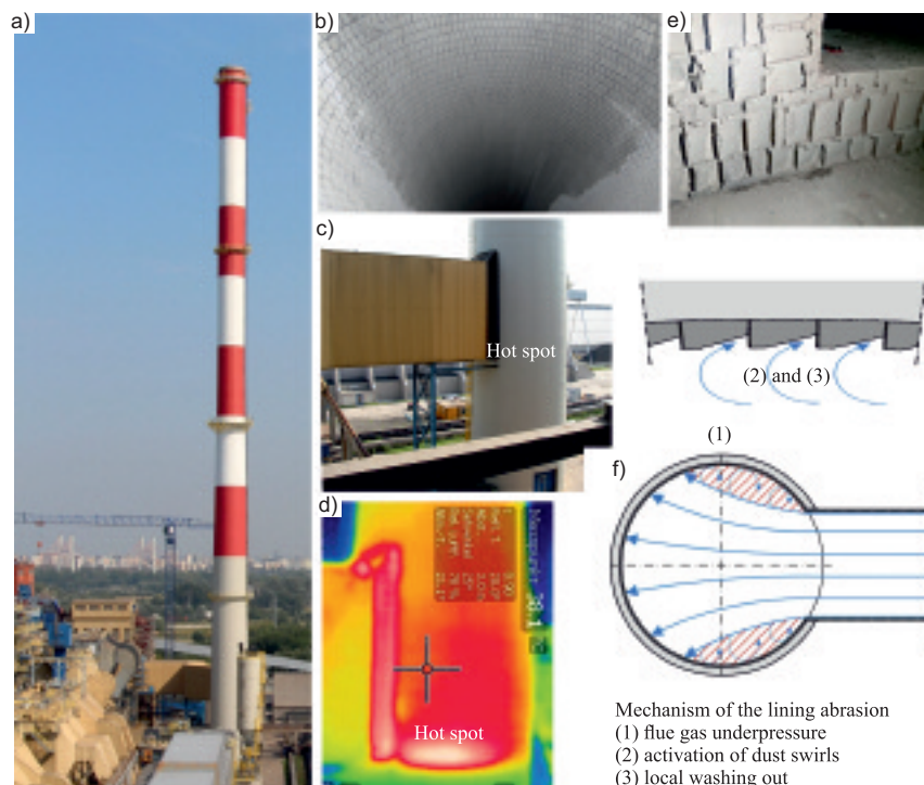
Photo 2. Chimney Siekierki: a) view on the NCD Chimney; b) flawless surface of the regular Pennguard™ lining; c) view on the external duct area; d) thermo-vision photo with a hot spot due to a local lining abrasion; e) view on the lining surface at the duct with visible lining abrasion; f) explanation of the local and partial lining abrasion
